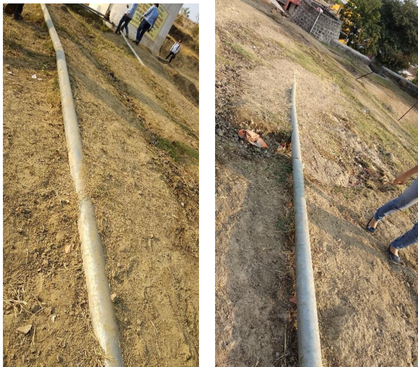
Figure 8.6.6F: Distribution network laid on ground
