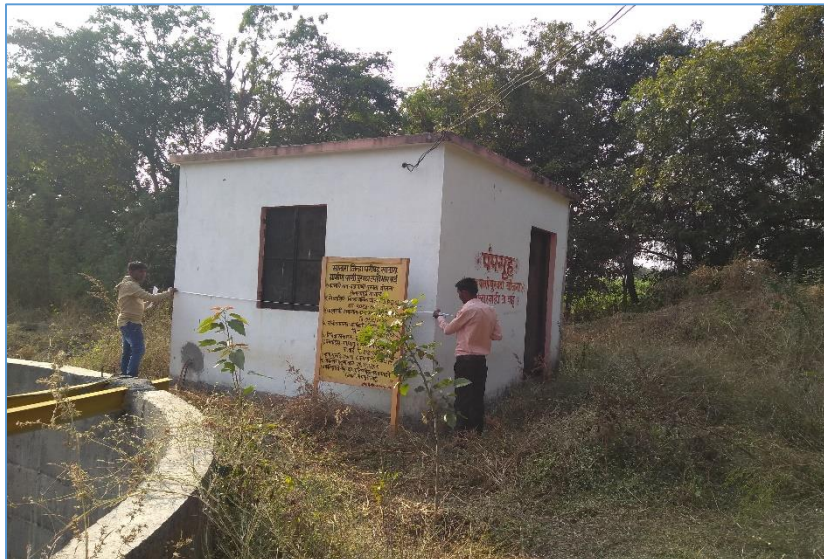
Figure 8.6.6C: Outside view of pump house
